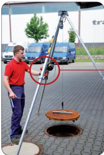
lifting of manhole-cover in connection with a tripod
